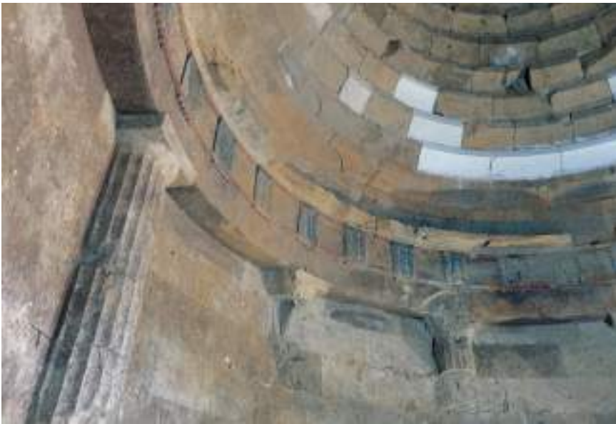
Fig. 16. The semi-columns in the central chamber of the Thracian cult building under the Chetinyova Mound near the village of Starosel. Photo: A. Sarbova
