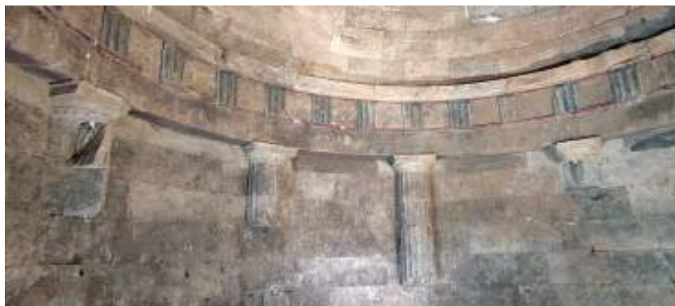
Fig. 10. The frieze with triglyphs and metopes in the sub-mound Thracian cult building near the village of Starosel. Photo: A. Sarbova
